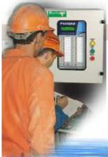
**TECHTROL WATER INGRESS DETECTION SYSTEM** FOR BULK CARRIERS
